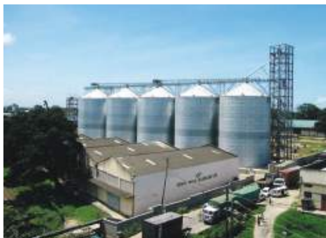
Custom-designed, manufactured and constructed cereal grain silos are the secret to success in maintaining mycotoxin-free stored grain prior to the feed manufacturing stage. (Image: Bentall Rowlands)
