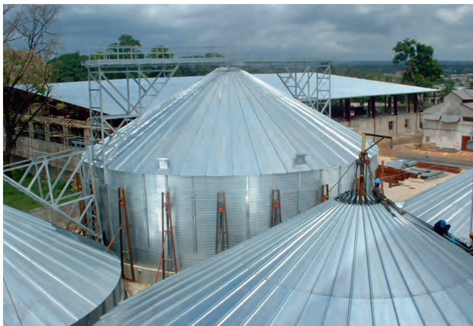
Custom-built grain silos are the key to the successful and safe storage of cereal grain.
