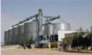
from grain silos
