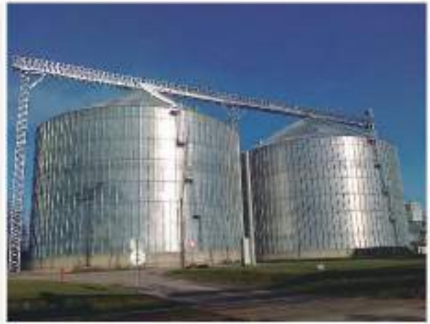
Diameter: 41,5 m - Capacity: 26.830 T - Total capacity: 54.000 T
