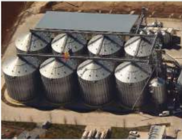
Diameter: 16,81 m - Capacity: 3.395 T - Total capacity: 21.000 T
