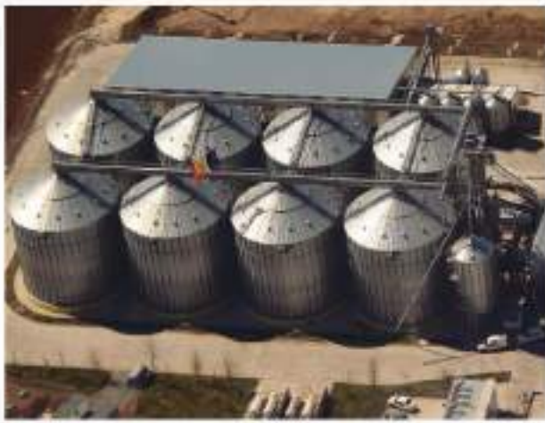
Diameter: 16,81 m - Capacity: 3.395 T - Total capacity: 21.000 T
