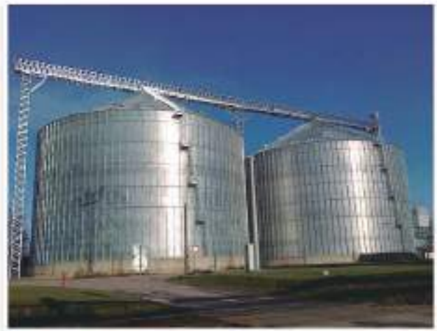
Diameter: 41,5 m - Capacity: 26.830 T - Total capacity: 54.000 T
