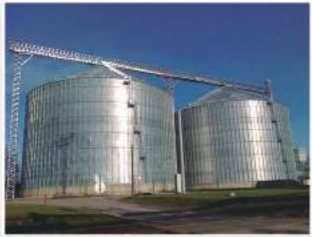
Diameter: 41,5 m - Capacity: 26.830 T - Total capacity: 54.000 T
