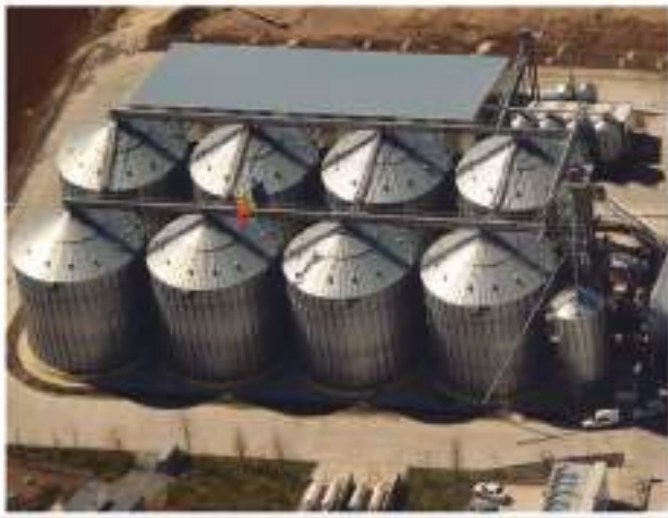
Diameter: 16,81 m - Capacity: 3.395 T - Total capacity: 21.000 T
