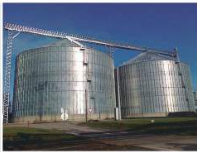
Diameter: 41,5 m - Capacity: 25,830 T - Total capacity: 54,000 T
