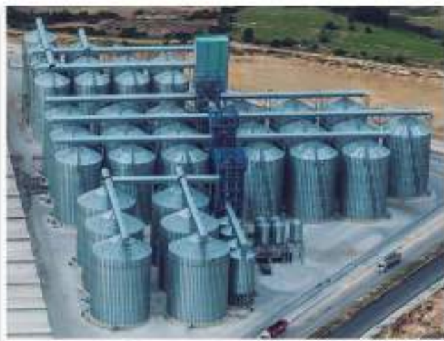
Diameter: 18,33 m - Capacity: 5,333 T / Diameter: 14,51 - Capacity: 3,300 T Total capacity: 200,000 T
