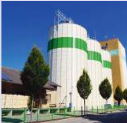
Bespoke Eurocode designed facility in Germany.
