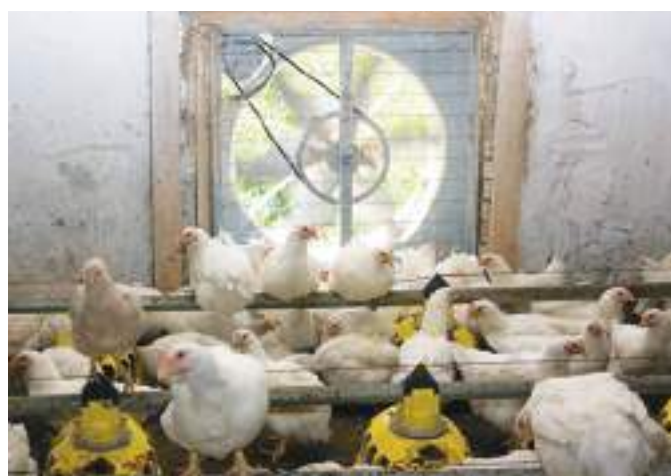
It is essential to properly maintain all house ventilation equipment and accessories. (Image: Poultrysite)
