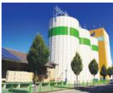
Bentall silo barrels utilise 100mm of pitch of corrugated steel, which adds strength and helps reduce product hang-up.
