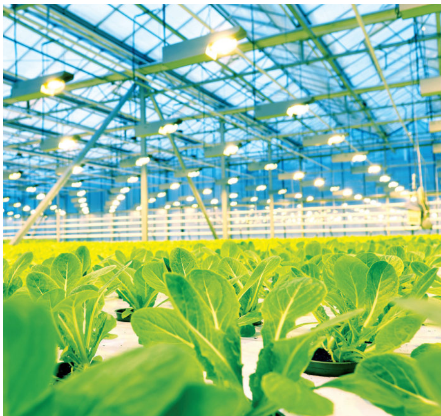
LaaP eliminates local ballast equipment on each fixture from the growing area.
